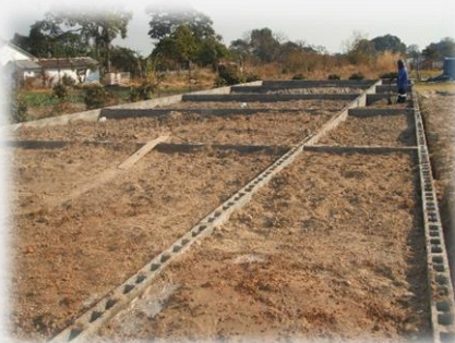
Filling in the foundations to level the building
