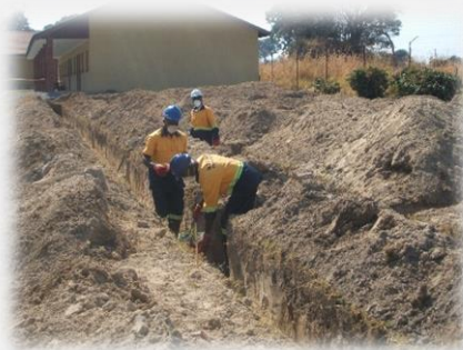
Digging the trenches ready to lay the foundations
