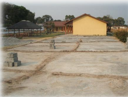
Slab complete ready for the walls to go up
